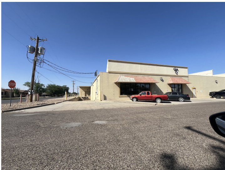
LOADING DOCK FOR 7,907 SF SUITE
