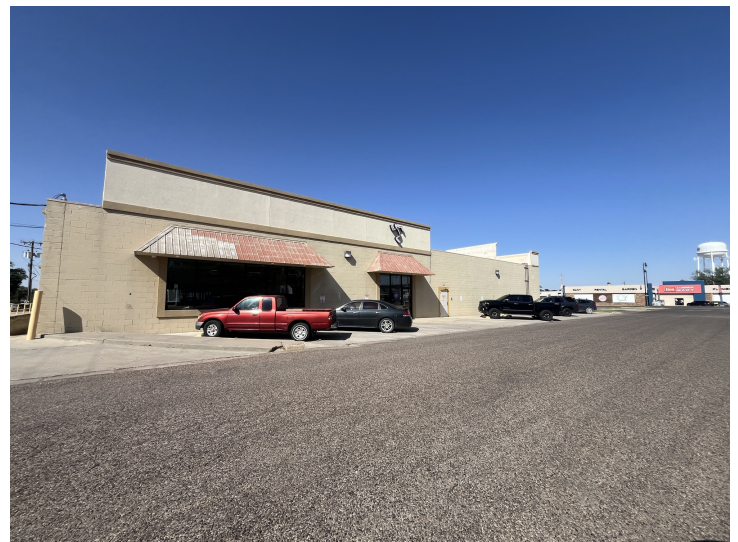
SOUTHERLY SIDE OF BUILDING, ANGLED PARKING
